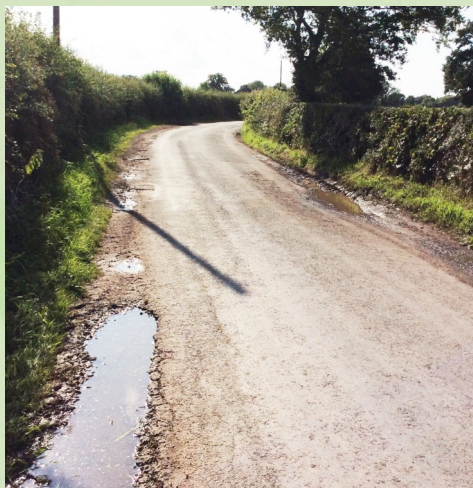
Bad potholes and degradation on Lodmore Lane
